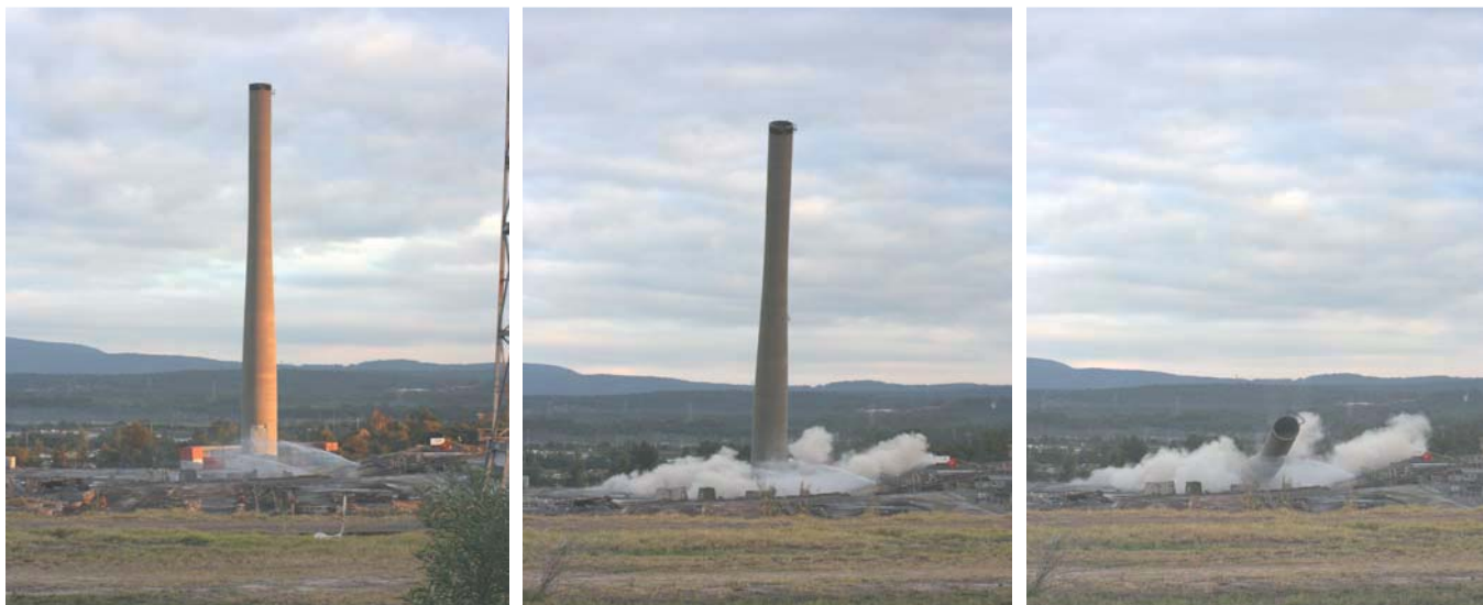
Figure 2: Demolition of the large concrete stack
